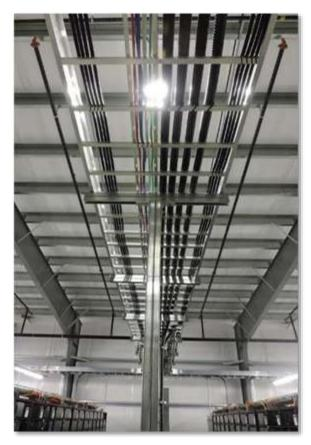
Figure 11: System Cable Tray -1
